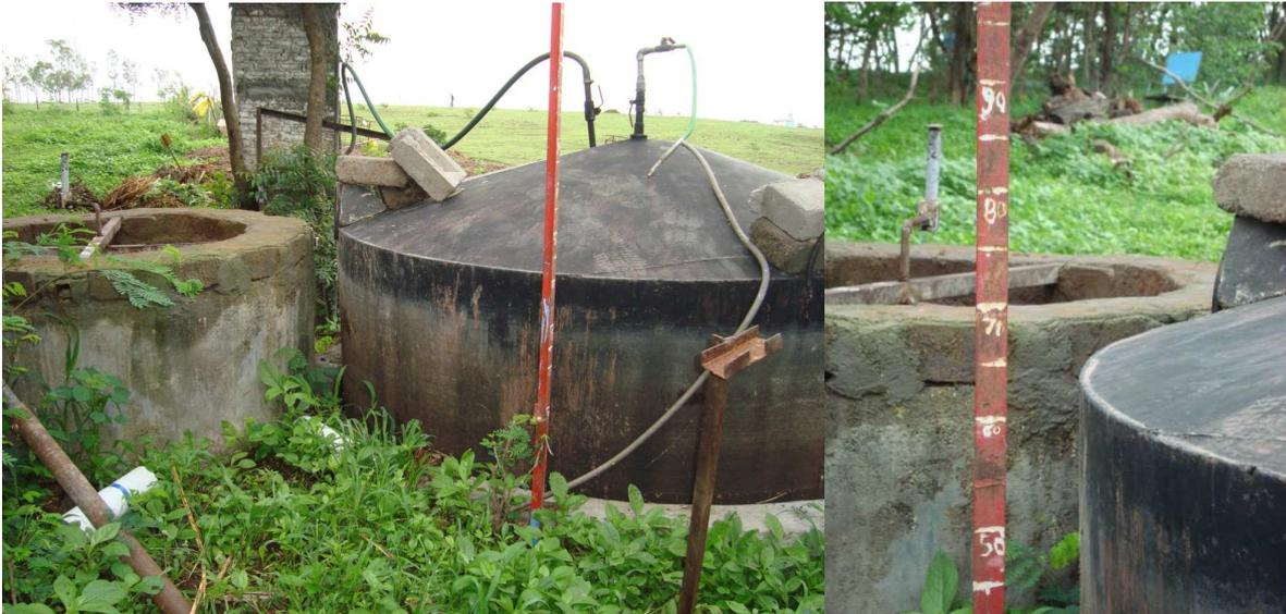
Using the measuring stick next to the gas holder note down the reading before and after every feeding, and enter these numbers into columns 4 and 5.
